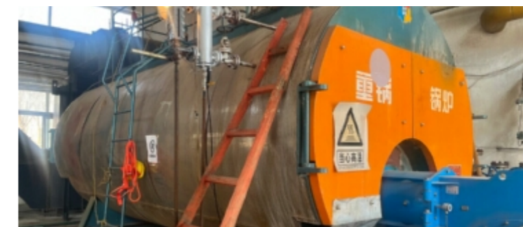
Boiler tube pickling
